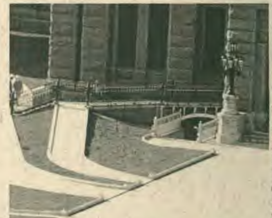
Ramps under construction at the Capitol.
