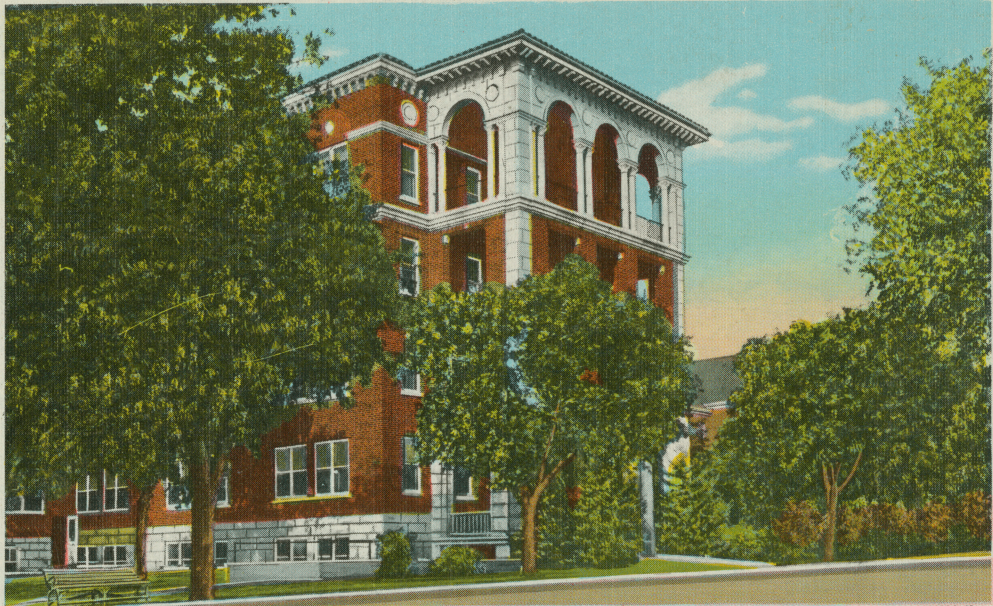
Terrell State Hospital, Terrell, Texas
